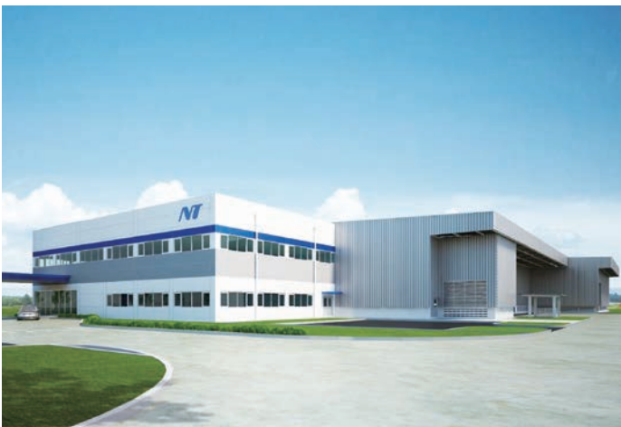
INDONESIA OFFICE / FACTORY
